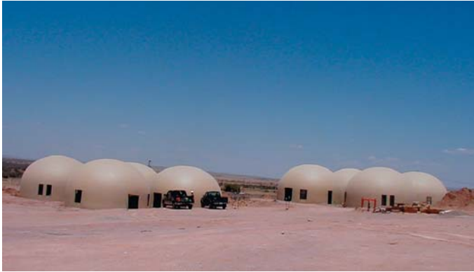
TOLCHI KOOH INC. (TOLANI LAKE, AZ) 2003 38' Diameter by 22.5' High School Teacher Housing - 24 Domes
