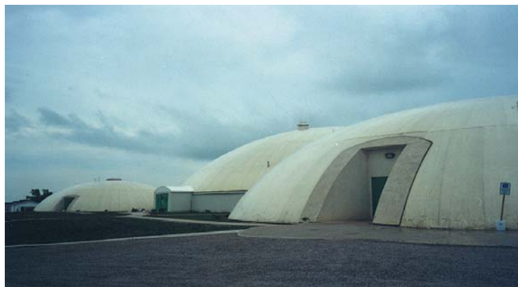
PATTONSBURG R-II SCHOOL DISTRICT (Pattonsburg, Mo) 1997 110' Diameter by 27.5' High 150' Diameter by 47' High Classrooms and Gymnasium - 4 Domes
