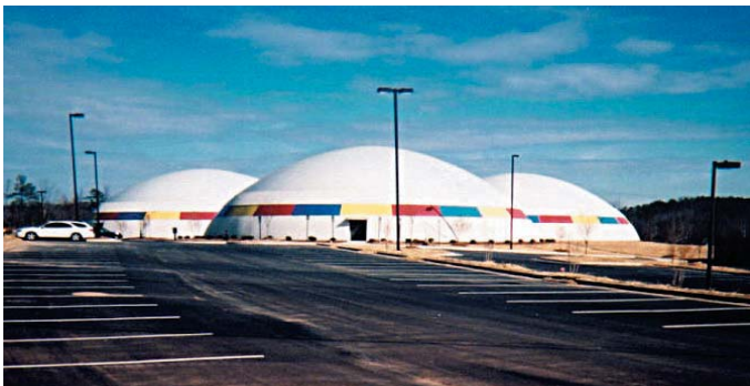
NORTH CAROLINA SCHOOL OF COMMUNICATION ARTS (RALEIGH, NC) 2003 118' Diameter by 34' High - 3 Domes
