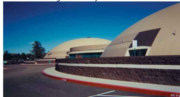
CRADLEBOARD ELEMENTRY SCHOOL (Whiteriver, Az) 120' Diameter by 30 High 110' Diameter by 27' High Classrooms and Gymnasium - 3 Domes
