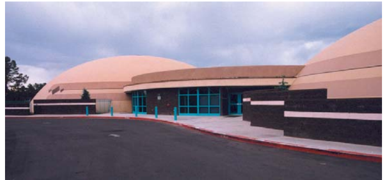
PAYSON UNIFIED SCHOOL DISTRICT (Payson, Az) 120' Diameter by 42 High 200' Diameter by 50 High Elementry School and High School Gymnasium - 4 Domes
