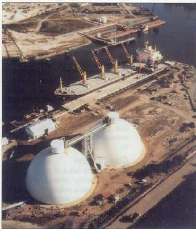
Cement storage domes for North Texas Cement - Houston, Texas.
