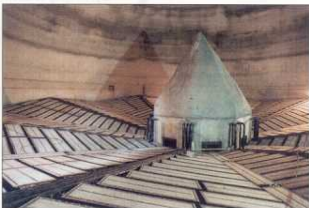
Inside the dome silo - segmented fluidised bottom. Left - side view, right - viewed from top of dome.
