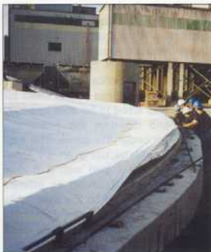
Figure 1 (left). Inflated air form. Figure 2 (right). Attaching air form to the foundation.
