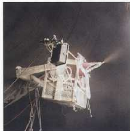
Figure 5. Spraying shotcrete embedding rebar.
