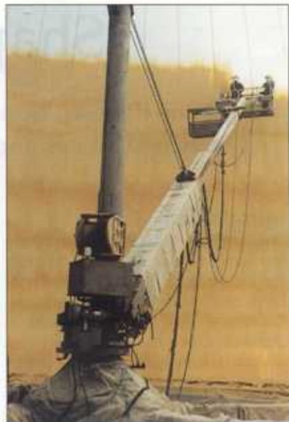
Figure 4. Spraying polyurethane foam.
